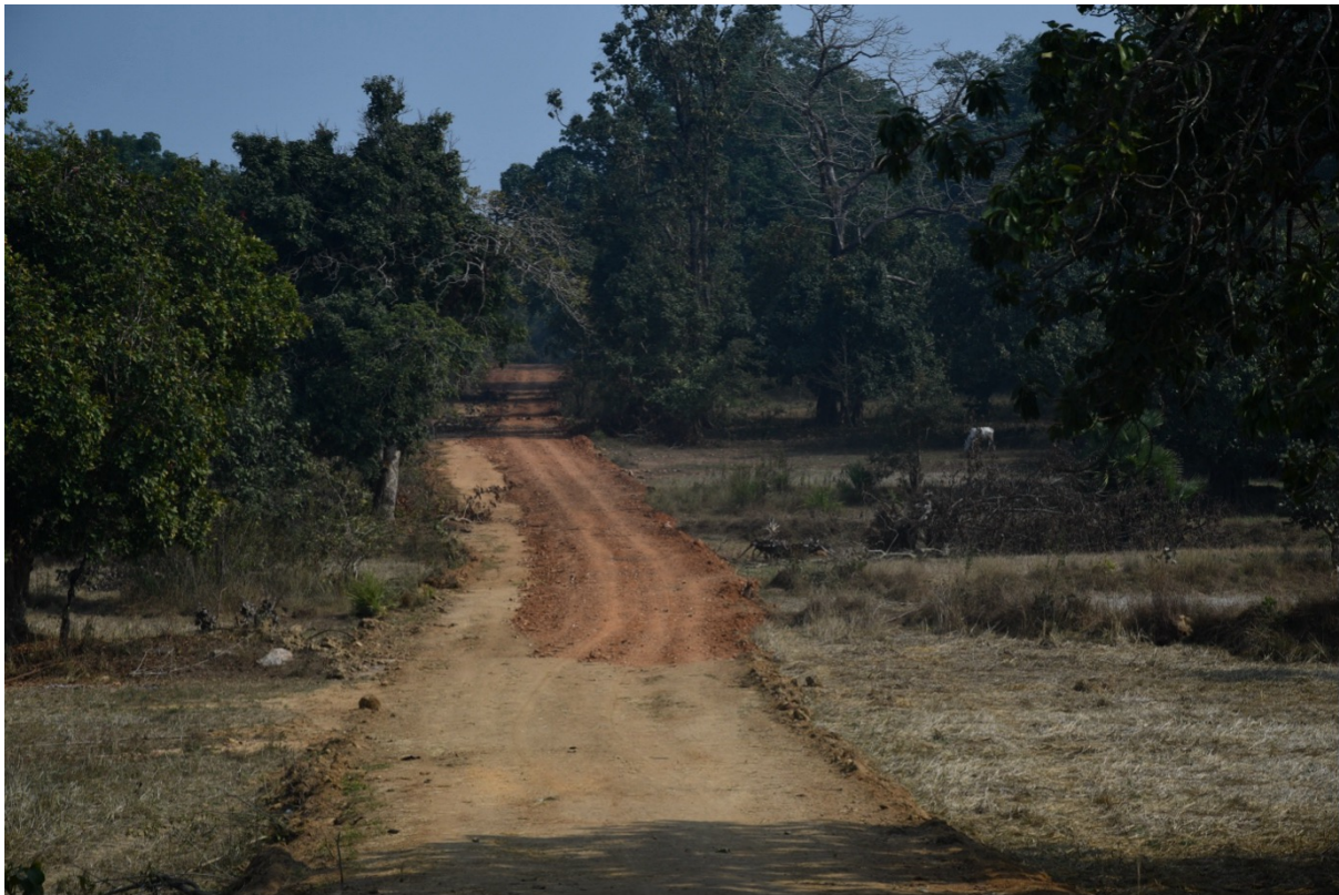
Figure 13: Road at Burji village, this road is being laid from Gangaloor to Nelasnar
