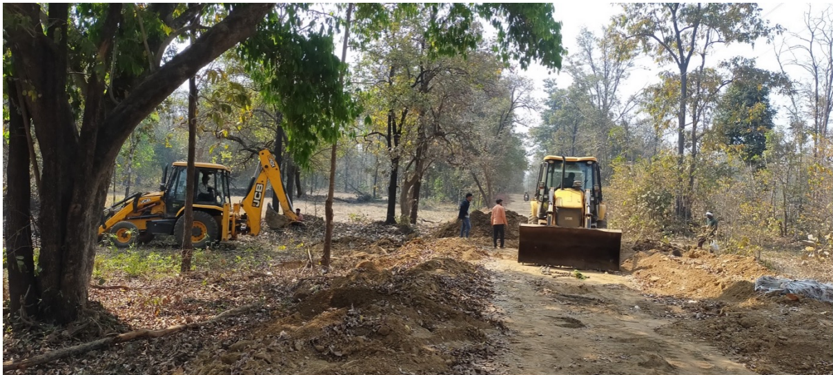
Figure 22: Road construction near Chilparas
