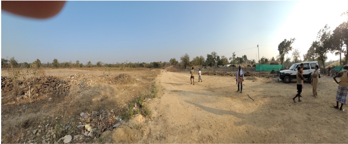
Figure 9: Silger camp 2 clearing area
